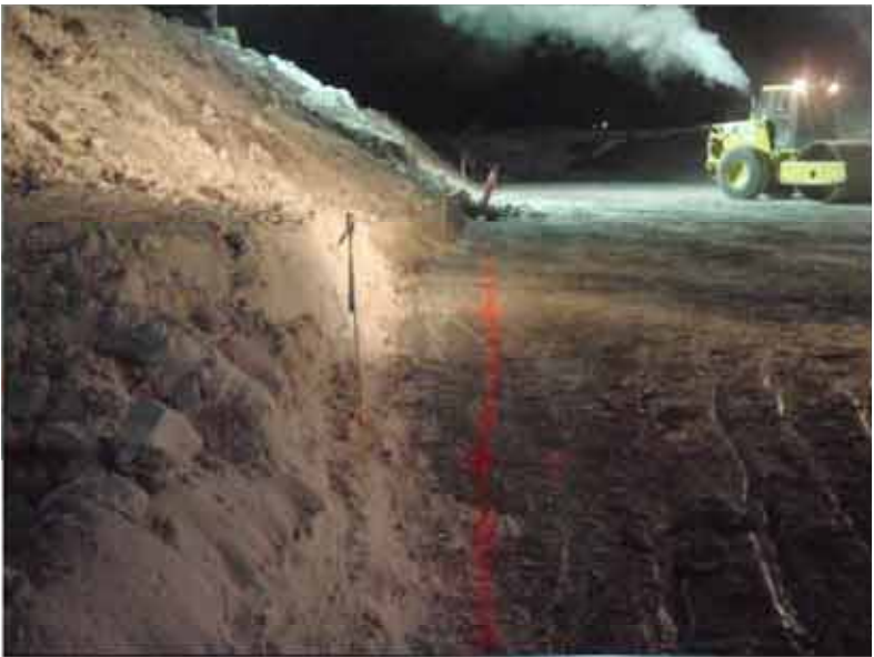
Photo 12: View from ~Sta 1+40 towards the central area of the key trench. Note that 5/8” material removal from 0+60 to 1+40 was approved today for placement
