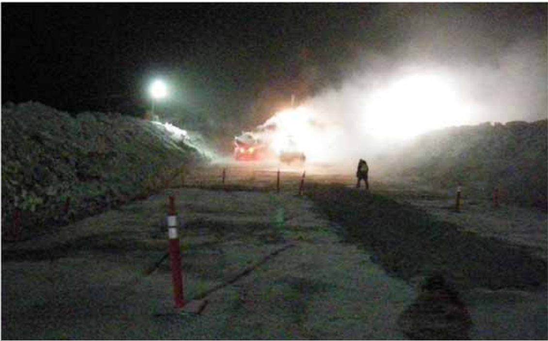
Photo 18: Material placement during the night shift. Looking north along the key trench. The delineators near the person mark the edge of the FCM placed during the day shift and the start of the material placed during the night shift.
