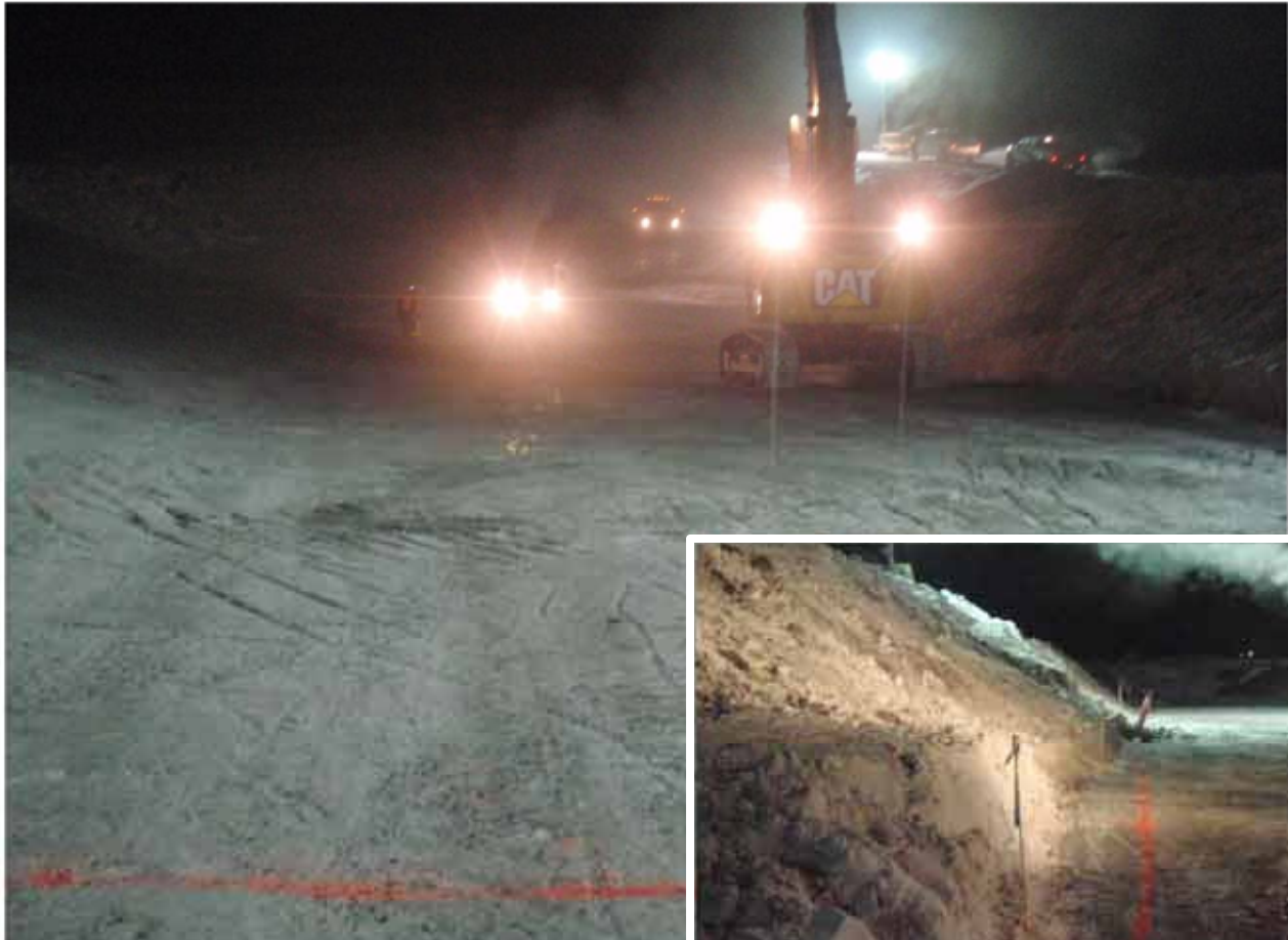
Photo 12: View from ~Sta 1+40 towards the central area of the key trench. Note that 5/8” material removal from 0+60 to 1+40 was approved today for placement
