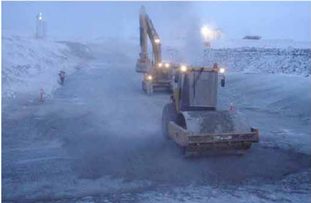
Photo 10: ~E view of vibrator compactor static rolling saturated FCM around station 0+85.
