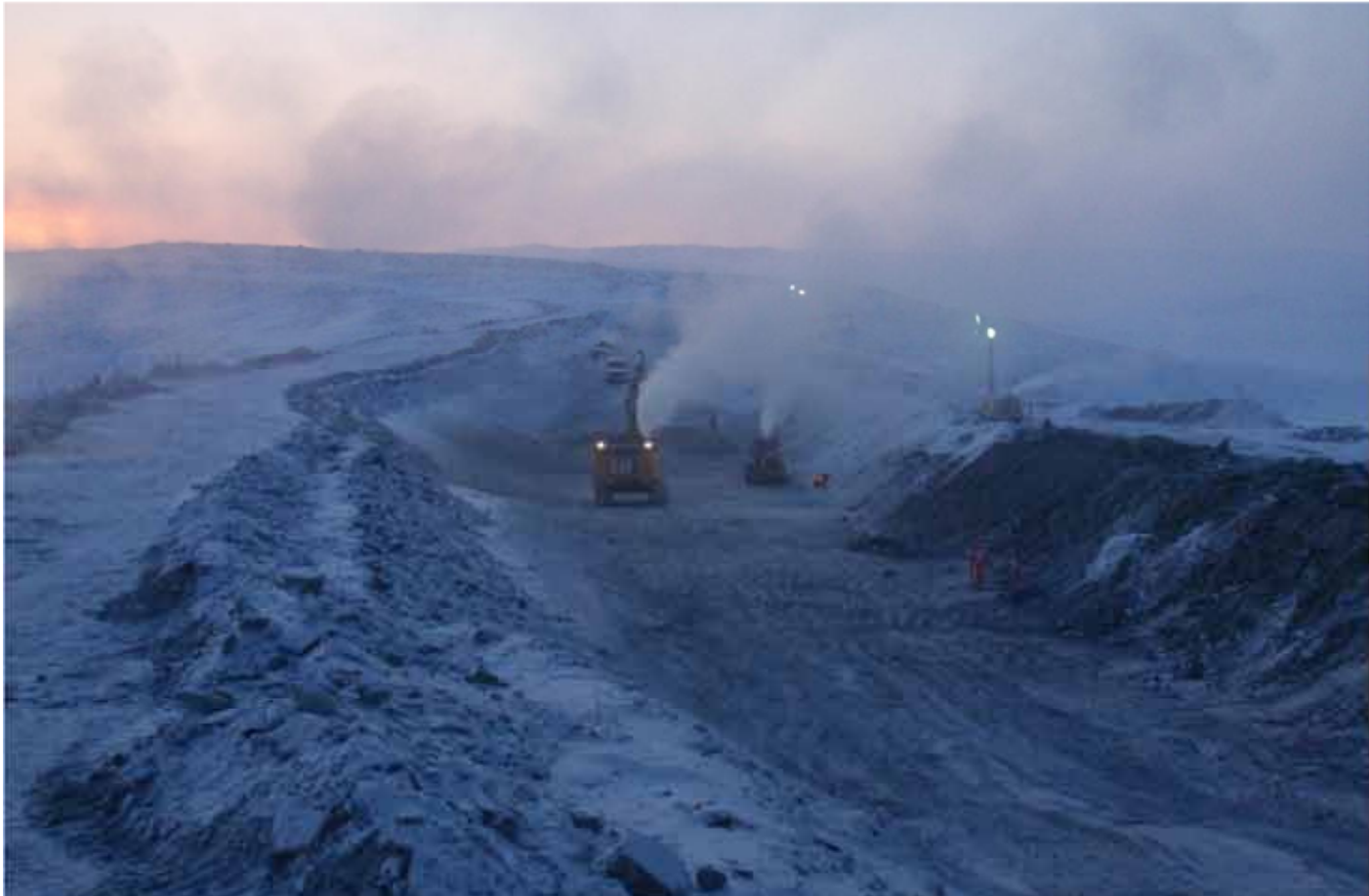
Photo 9: ~ ESE view down key trench. Note the 345 excavator and bobcat cleaning the central key trench area in preparation for the afternoon placement.
