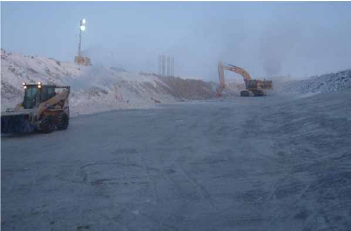
Photo 1: ~ NE view down key trench of cleaning activities. Note the excavation cleaning the DS slope around station 1+50.
