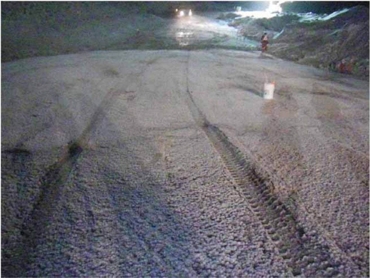
Photo 15: Pickup tracks across the fresh (not frozen back) FCM placed during the dayshift.
