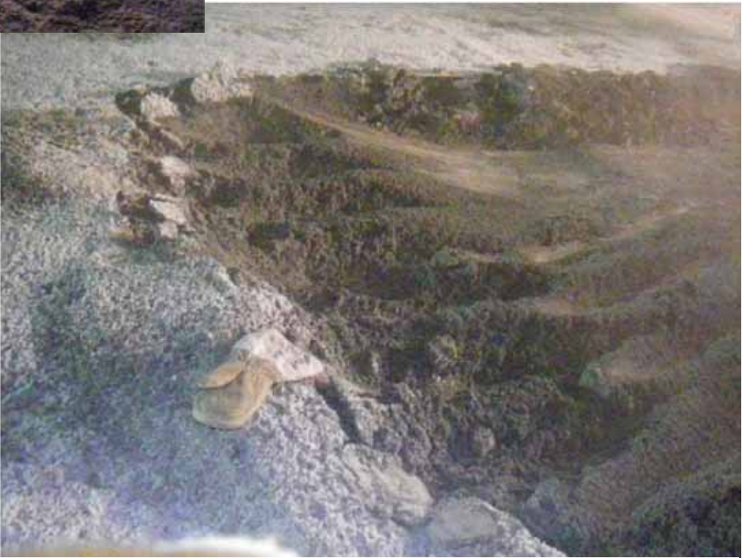
Photo 17: Edge of material being removed by CAT 345 excavator, as only the toothed bucket was available some ridges of material remain.
