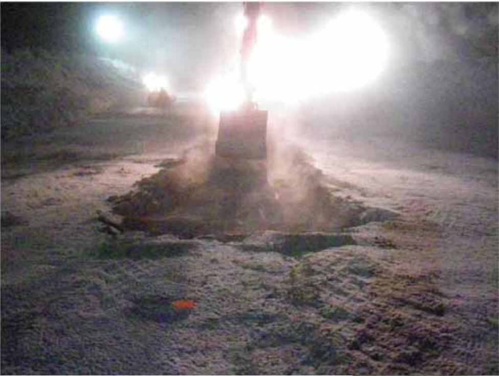
Photo 16: CAT 345 excavator removing damaged frozen core from pickup truck tracks.
